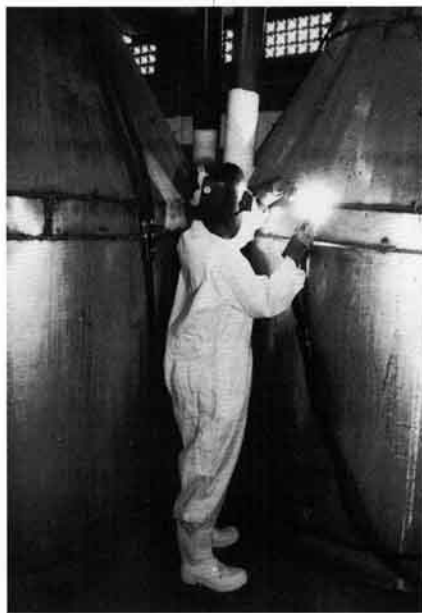
A welder puts to work on one of the cylindro-conical fermenters.
