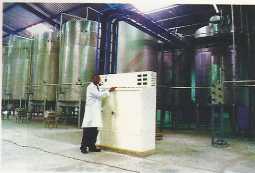
Winani Chiwowa, head brewer of Trade Kings, in its maheu plant while under construction.
